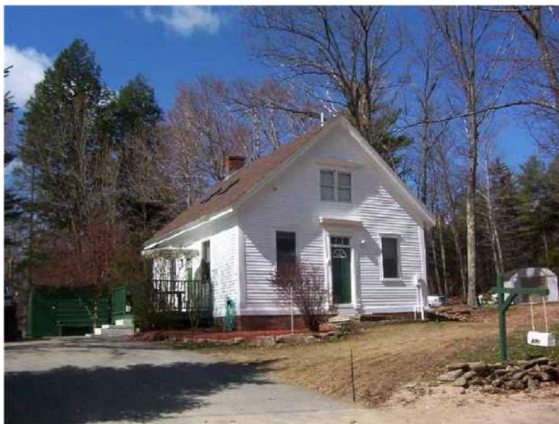
North Barnstead Schoolhouse
